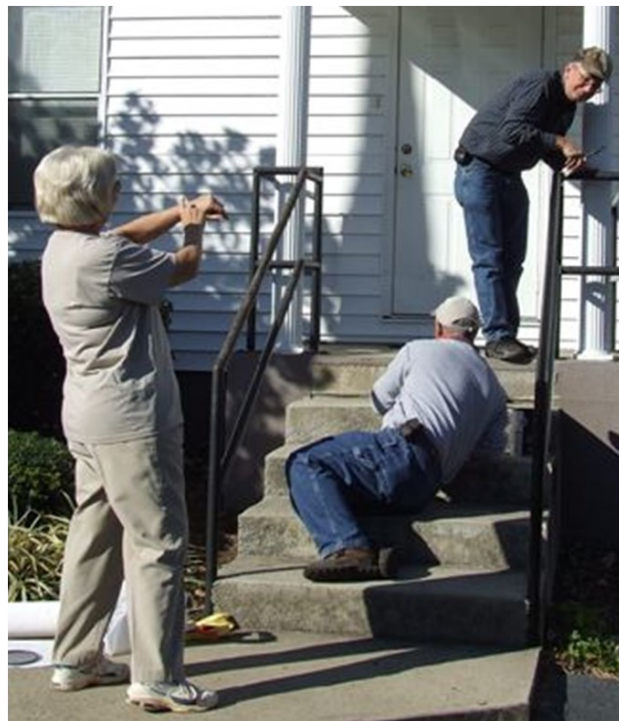
Pat Foy, tries to keep the workers on a schedule , but with these two, it might be hard, Keith Rimer on steps, Jack Mills on landing.
