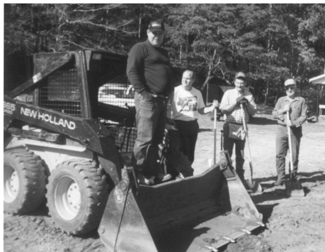
End of 1997- Decided to build a Fellowship Hall to be used as church When construction started on Church.
