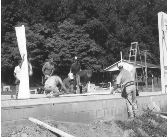
Summer through September 1999 Men and Women worked very hard to construct the Fellowship hall
