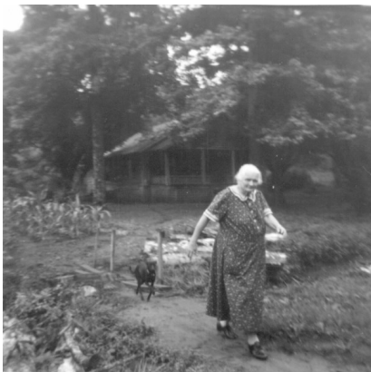
Carrie Ritchey on her way from her house to the construction site for Midway Baptist Church
